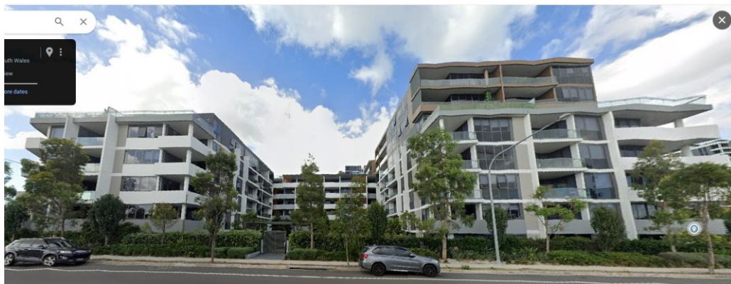
Existing flat building to the south within BATA 1 Precinct as viewed from Tingwell Boulevard
